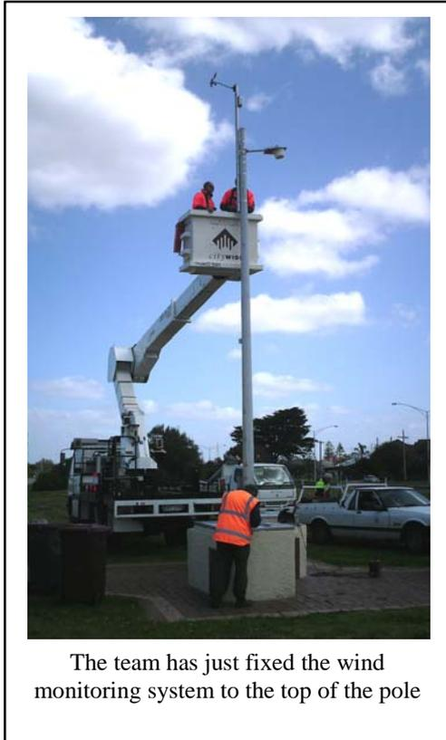
At the third site, a new mast structure was required with a purpose built housing for the logger unit.
